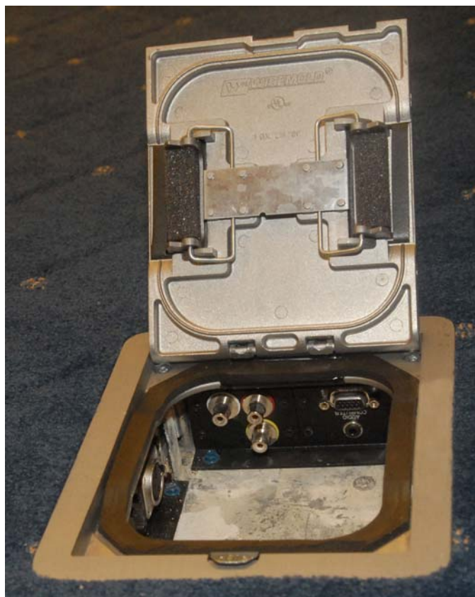
Figure 1. Computer and Audio/Video Connection Access in Floorbox
