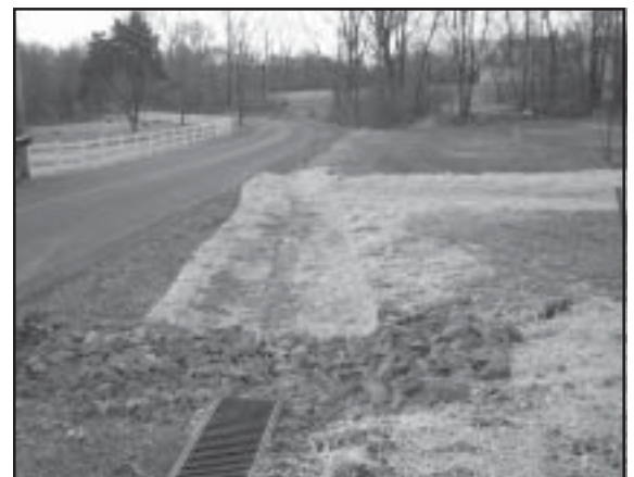
Install lining for better erosion control.
