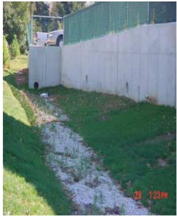
Infiltration trench captures stormwater runoff from the roof and parking lot. Beneath 6 inches of stone at the surface is an infiltration bed that temporarily stores stormwater prior to infiltration into ground below.
