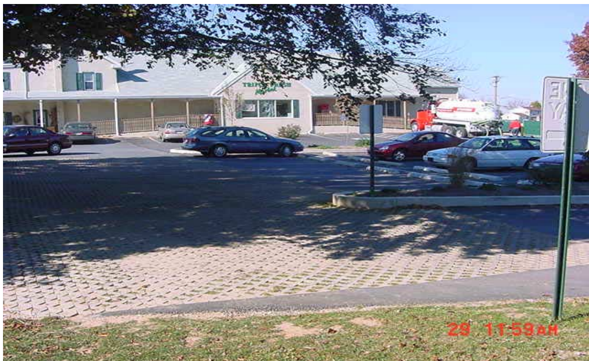
Brown colored paver blocks used to expand parking lot allow stormwater to seep into the ground and provide needed water for the roots of a large sycamore tree.
