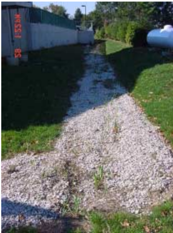
Infiltration trench captures stormwater runoff from the roof and parking lot. Beneath 6 inches of stone at the surface is an infiltration bed that temporarily stores stormwater prior to infiltration into ground below.
