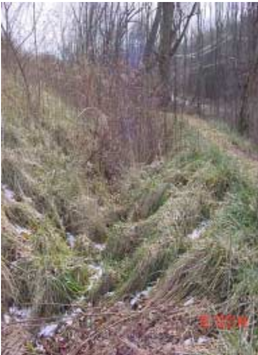
Narrow, vegetated recharge trenches follow land contours and take on a naturalized appearance.
