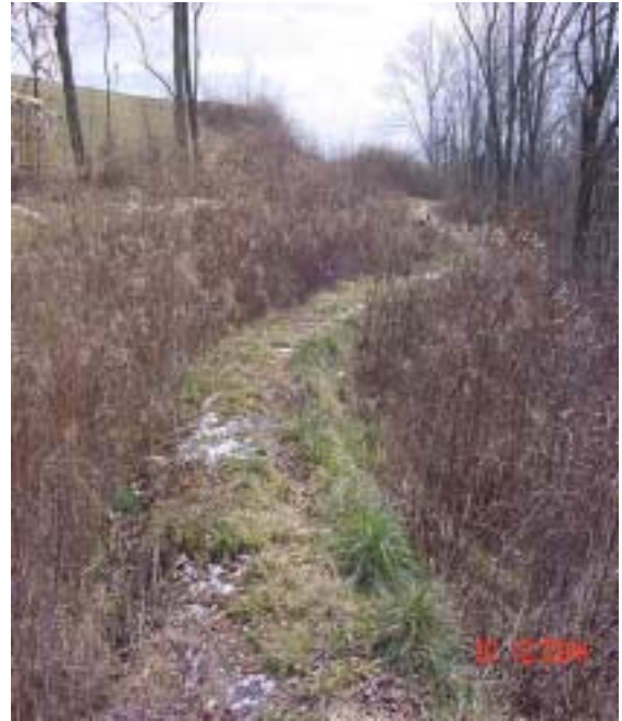
This grassy path is an embankment, or berm, creating depressions for recharge trenches located to the left of the path.
