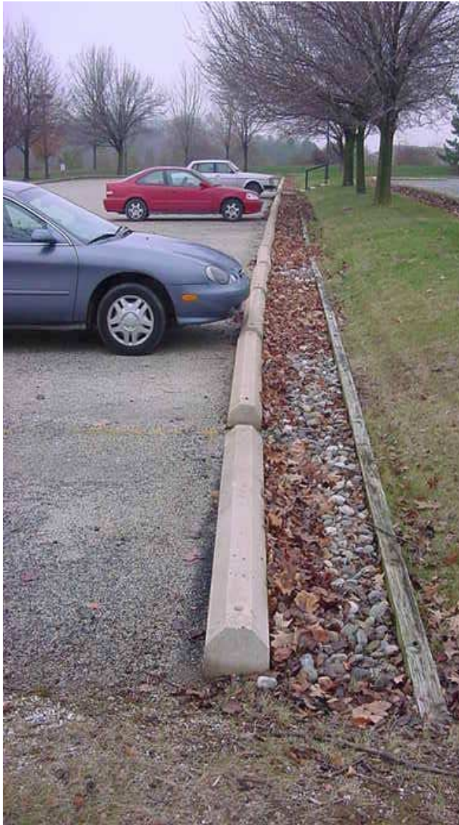
Along the edges of porous pavement parking bays are stone infiltration trenches that capture any runoff and enhance infiltration opportunities. (Parking bumpers allow runoff to be captured in stone infiltration trenches along parking lot edge.)
