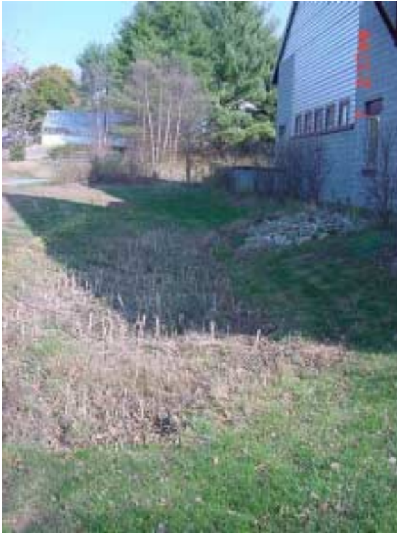
Vegetation in the Rain Garden (upper left) was cut back in the fall; rip rap bank along building receives runoff flowing directly off the roof. Upper right: downspout directs runoff into a grass-lined channel around cinder block wall. Below: Wetland vegetation thriving in and around wet pond pictured below.
