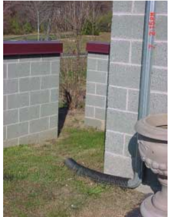
Vegetation in the Rain Garden (upper left) was cut back in the fall; rip rap bank along building receives runoff flowing directly off the roof. Upper right: downspout directs runoff into a grass-lined channel around cinder block wall. Below: Wetland vegetation thriving in and around wet pond pictured below.
