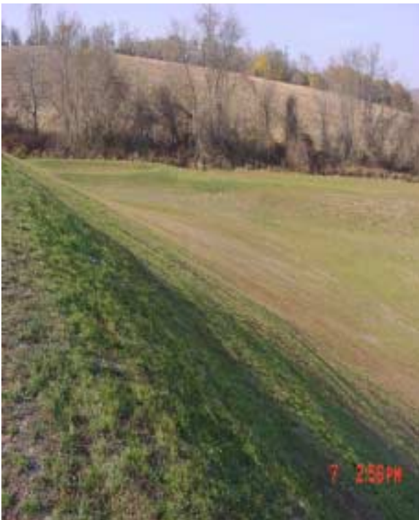
View of site infiltration basins.
