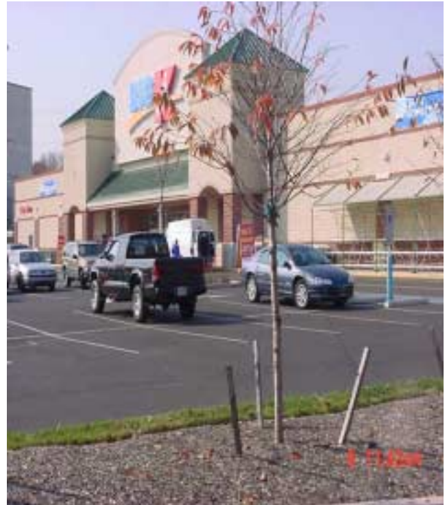
Stormceptors filter pollutants common in runoff from commercial parking lots (designed to capture “first flush”).
