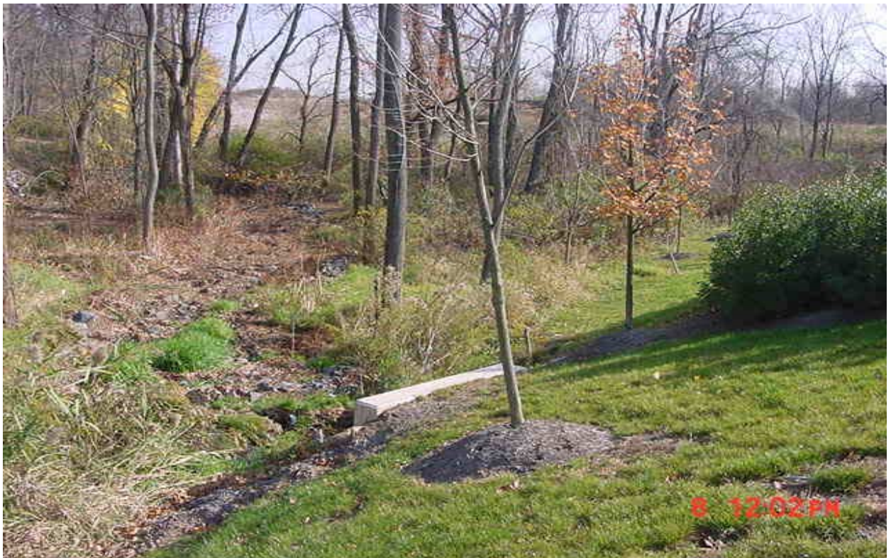
Wetland area behind site manages stormwater and provides riparian buffer for French Creek and wildlife habitat
