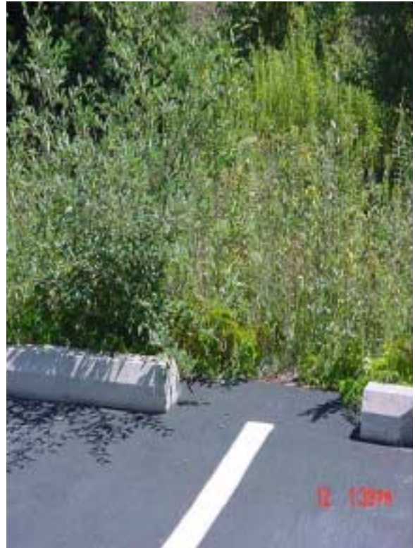
Pictured above: curbcut and parking bumpers direct parking lot runoff down a stabilized bank into the biofiltration swale. Biofiltration swales are well-vegetated, linear channels that filter pollutants in runoff through physical, chemical and biological actions of resident plants, soils and microbes. (gradual slope of less than 1% promotes slow flow of stormwater maximizing contact time with vegetation and soils.
