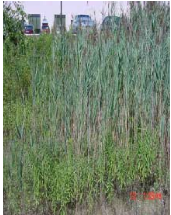
Pictured above: curbcut and parking bumpers direct parking lot runoff down a stabilized bank into the biofiltration swale. Biofiltration swales are well-vegetated, linear channels that filter pollutants in runoff through physical, chemical and biological actions of resident plants, soils and microbes. (gradual slope of less than 1% promotes slow flow of stormwater maximizing contact time with vegetation and soils.
