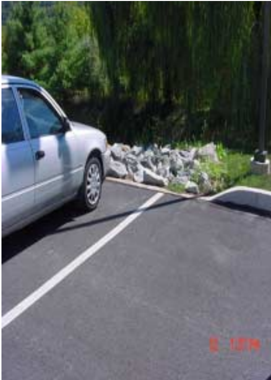
Pictured above: curbcut and parking bumpers direct parking lot runoff down a stabilized bank into the biofiltration swale. Biofiltration swales are well-vegetated, linear channels that filter pollutants in runoff through physical, chemical and biological actions of resident plants, soils and microbes. (gradual slope of less than 1% promotes slow flow of stormwater maximizing contact time with vegetation and soils.
