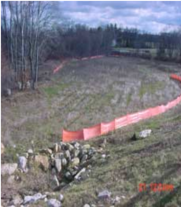
The vegetated swale is protecting this wetland mitigation area to prevent inundation during plant establishment.
