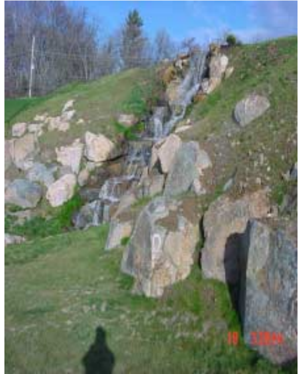
Pond water is pumped up to waterfall and returns to pond through grass swales enhancing aeration.
