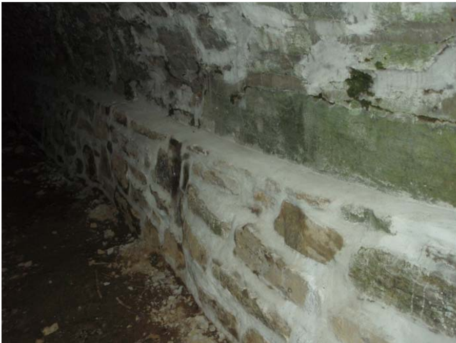
Chester Valley Trail Culvert #5 After
