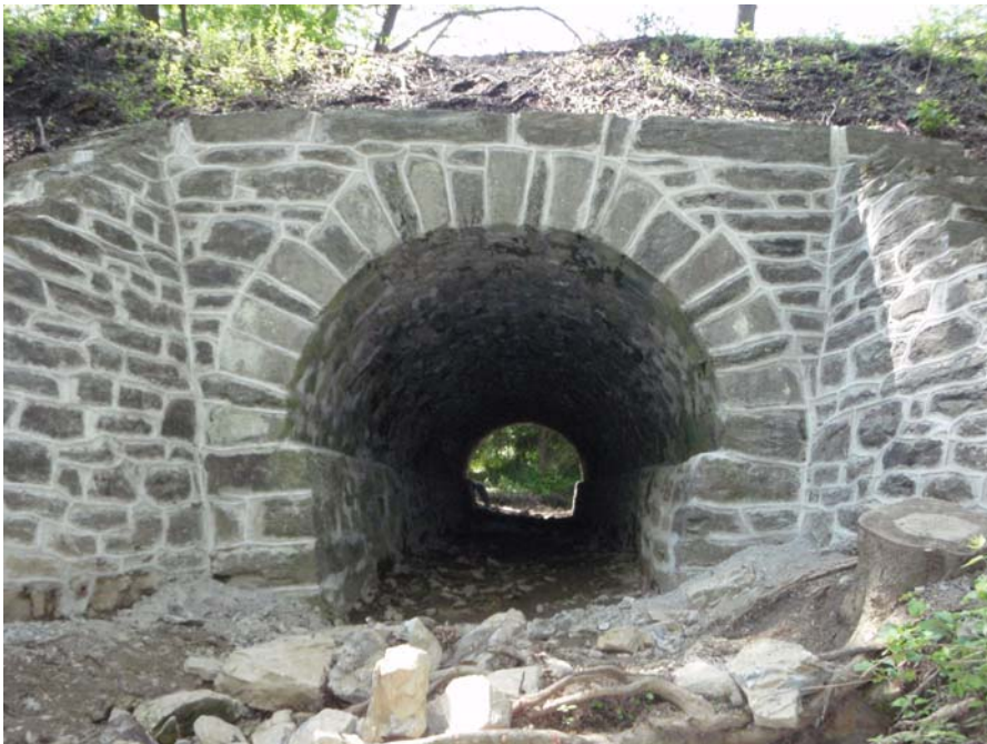
Chester Valley Trail Culvert #5 After
