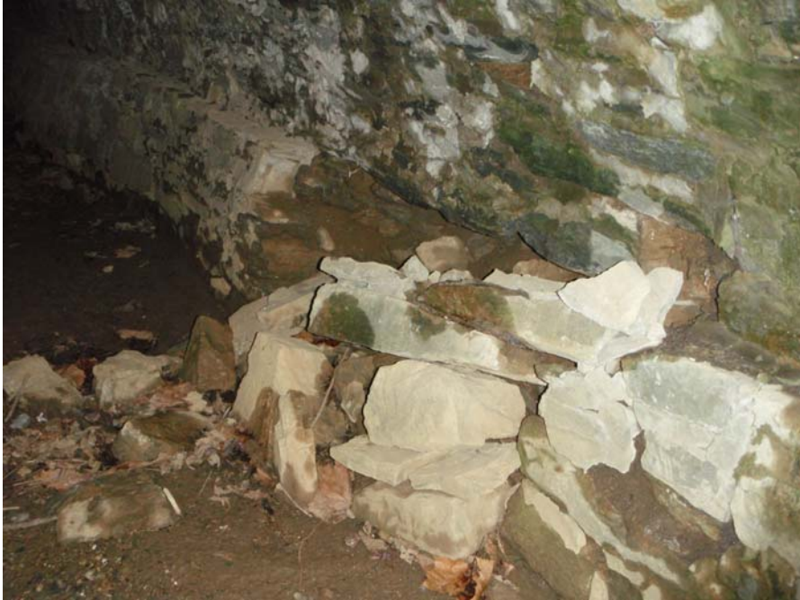
Chester Valley Trail Culvert #5 Before
