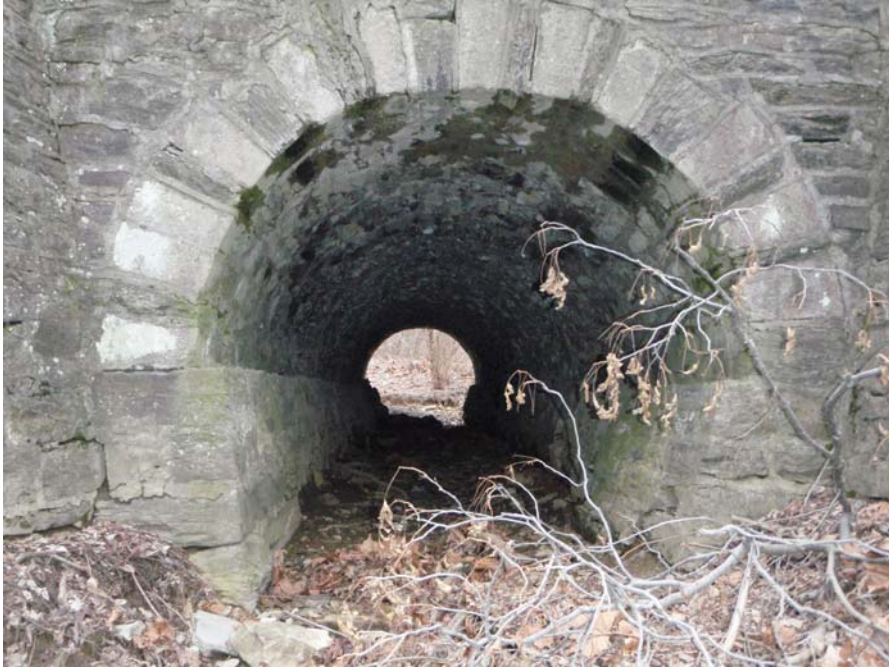
Chester Valley Trail Culvert #5 Before
