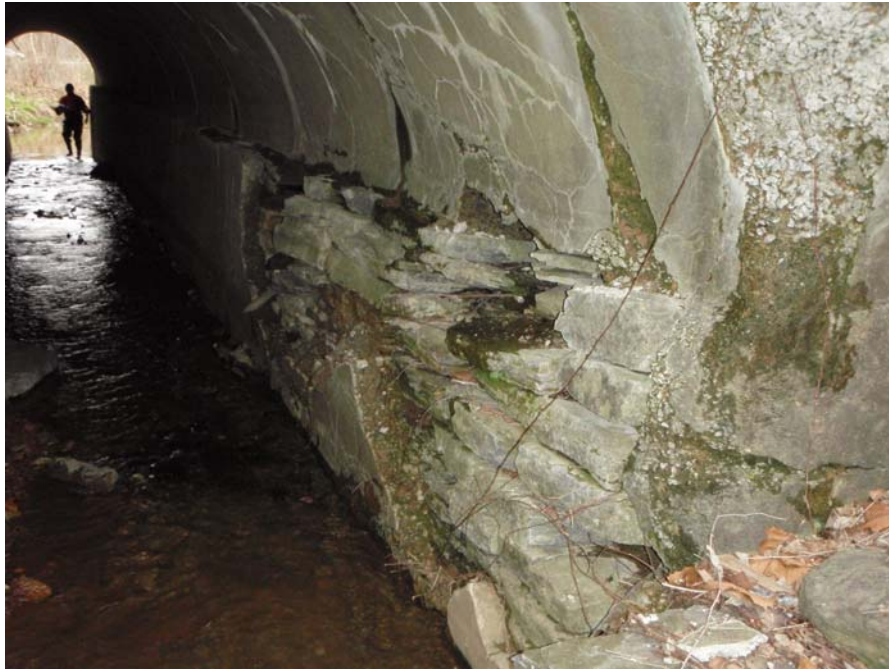
Chester Valley Trail Culvert #4A Before
