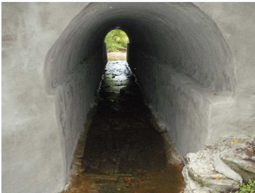
Chester Valley Trail Culvert #4A After
