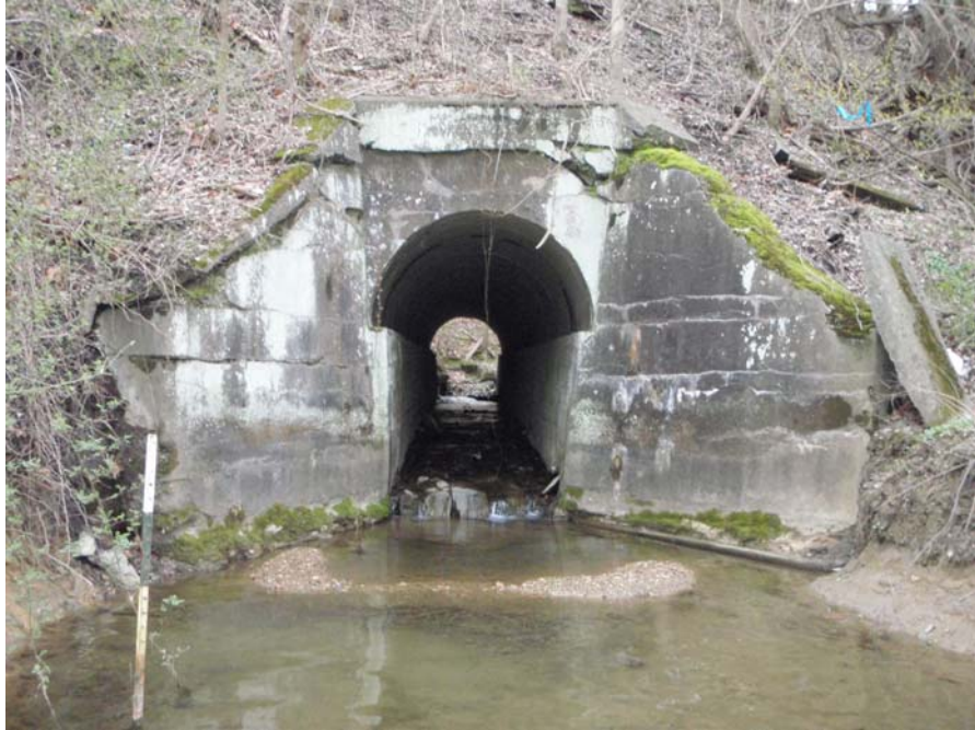
Chester Valley Trail Culvert #4A Before
