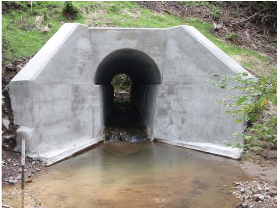
Chester Valley Trail Culvert #4A After
