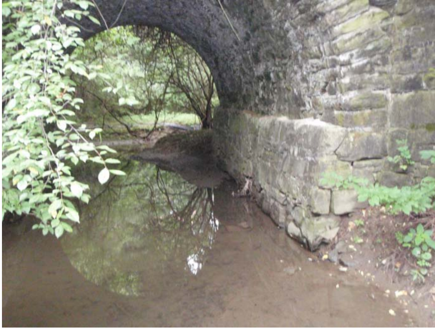
Chester Valley Trail Culvert #3 Before
