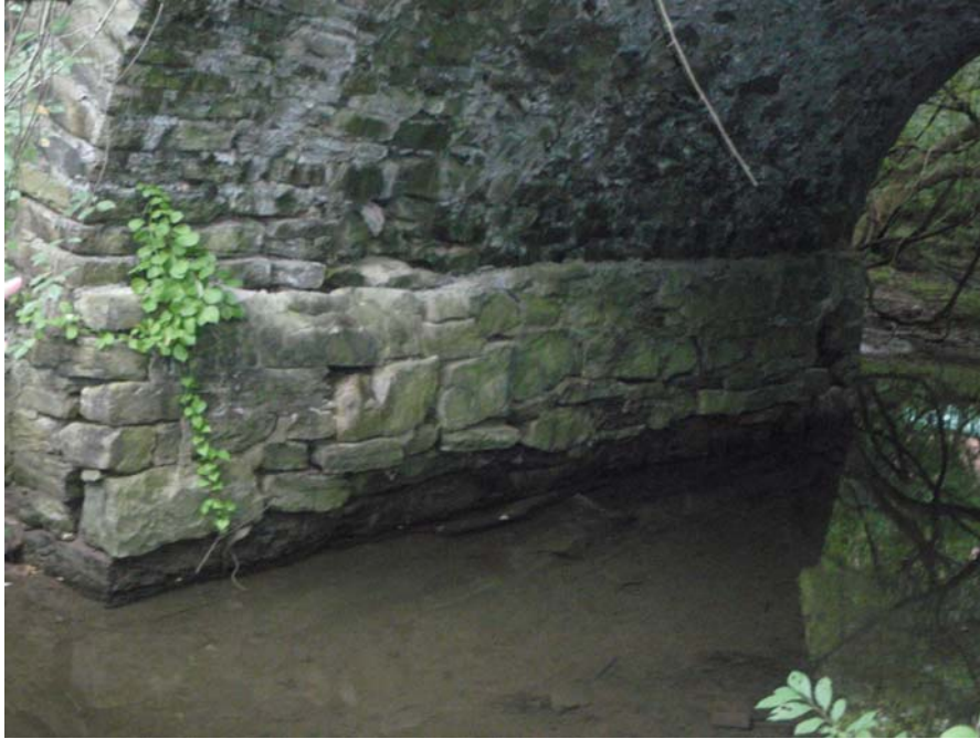
Chester Valley Trail Culvert #3 Before
