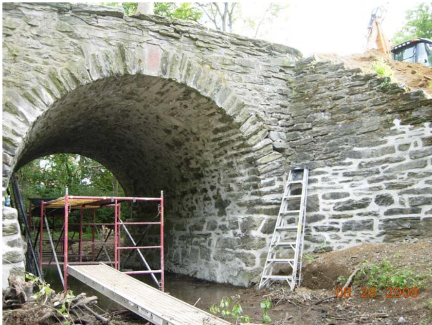
Chester Valley Trail Culvert #3 After
