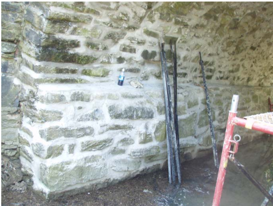
Chester Valley Trail Culvert #3 After
