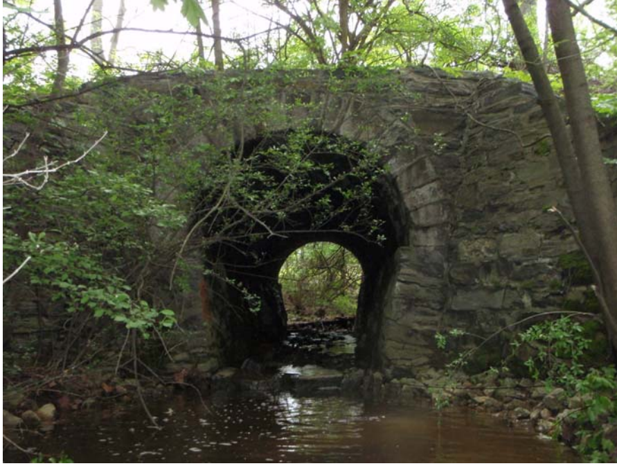
Chester Valley Trail Culvert #11 Before
