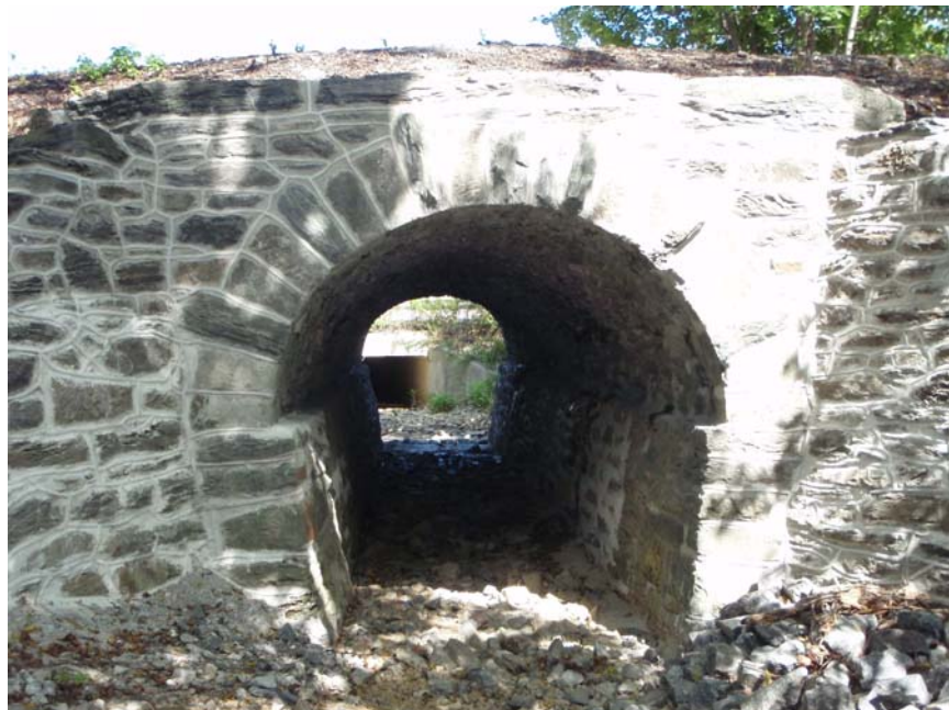
Chester Valley Trail Culvert #11 After
