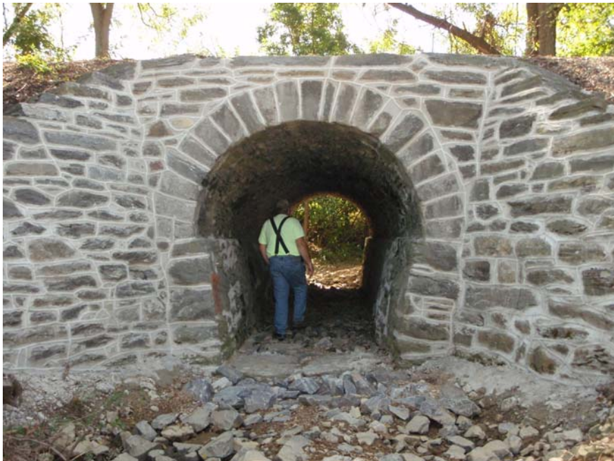
Chester Valley Trail Culvert #11 After
