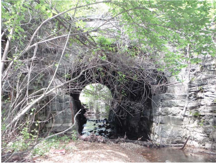
Chester Valley Trail Culvert #11 Before
