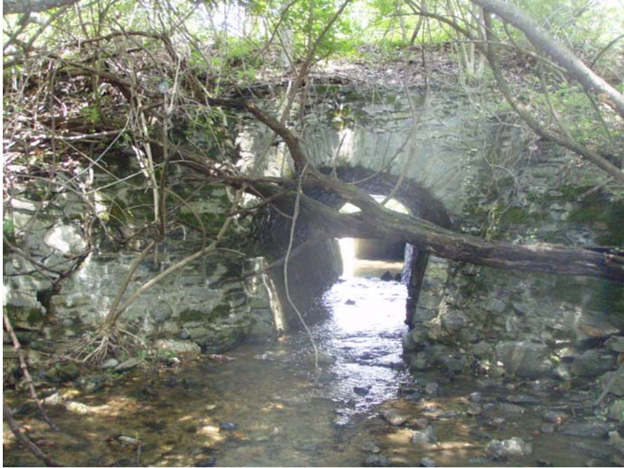
Chester Valley Trail Culvert # 10 Before
