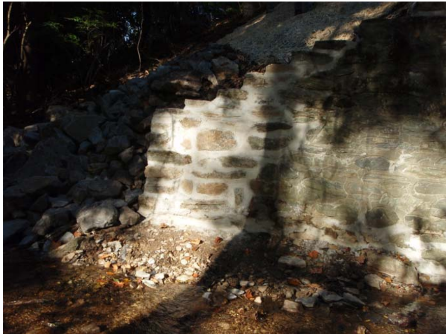
Chester Valley Trail Culvert #10 After
