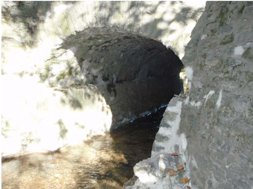
Chester Valley Trail Culvert #10 After
