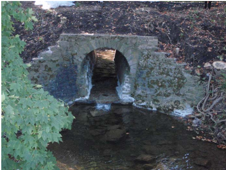
Chester Valley Trail Culvert #10 After
