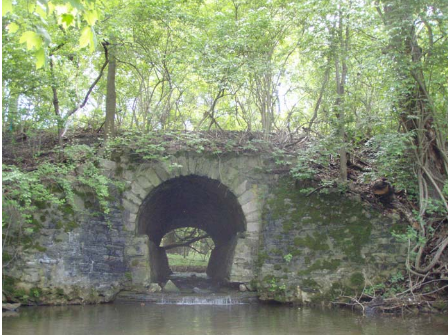
Chester Valley Trail Culvert #10 Before
