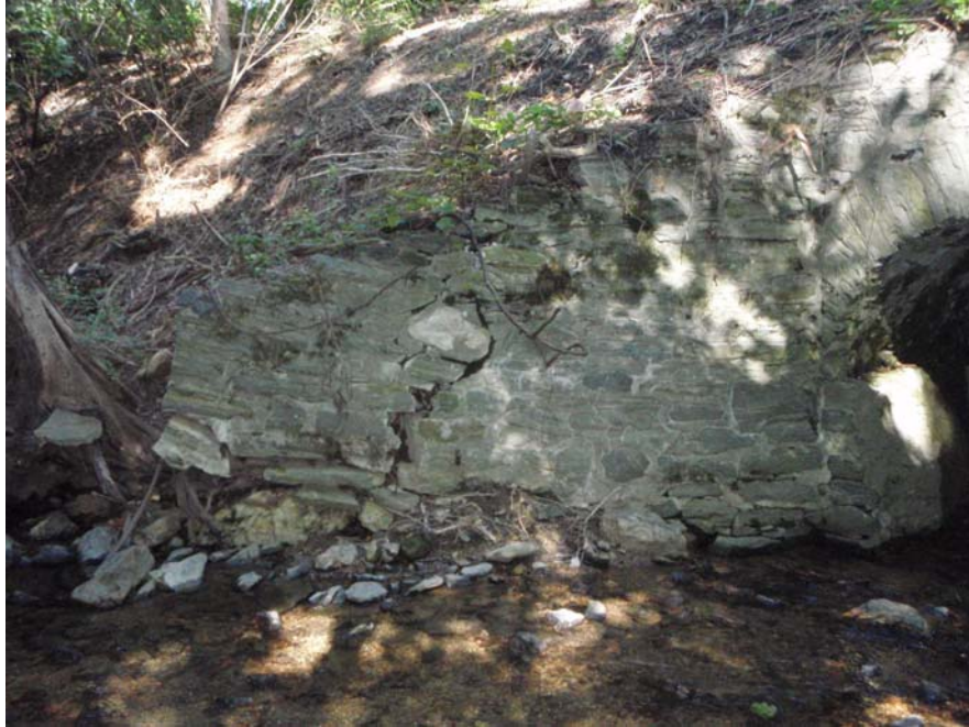
Chester Valley Trail Culvert # 10 Before
