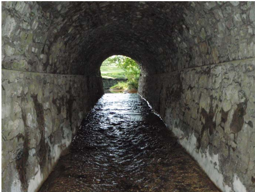
Chester Valley Trail Culvert #1 After
