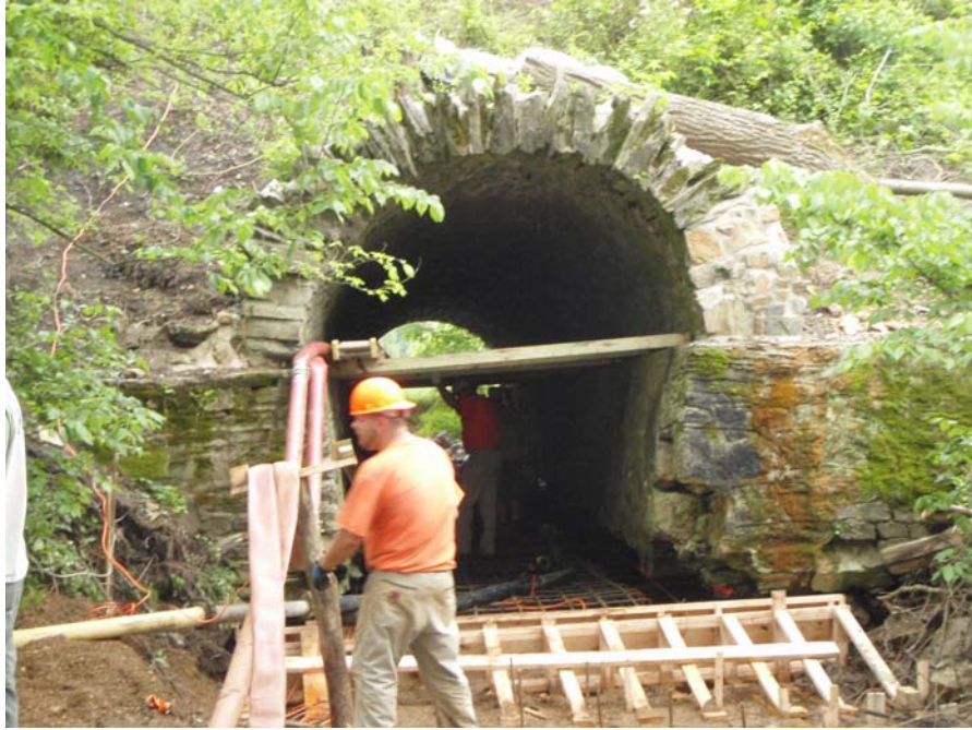
Chester Valley Trail Culvert # 1 Before
