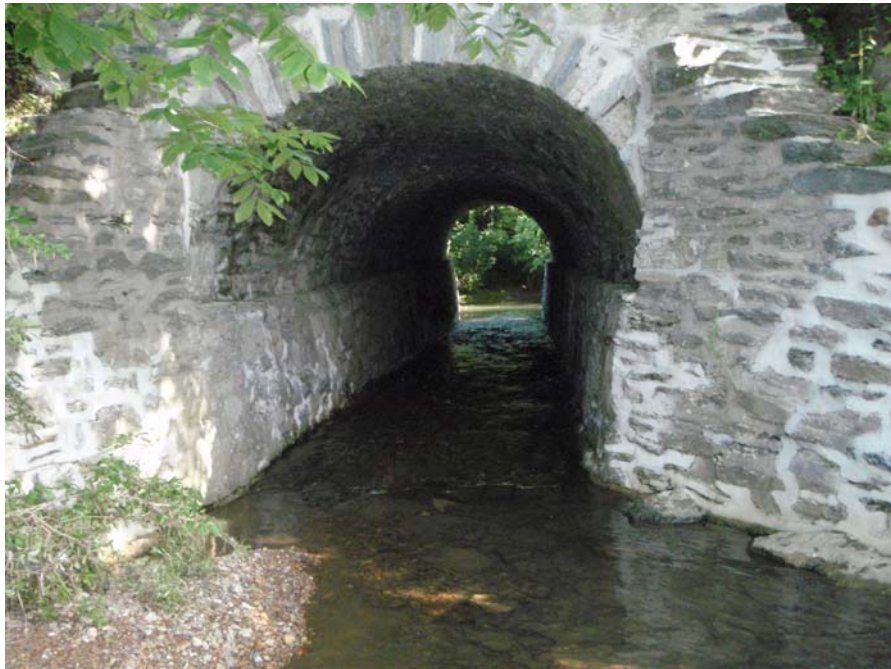
Chester Valley Trail Culvert #1 After
