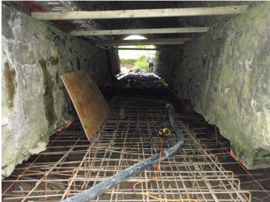
Chester Valley Trail Culvert #1 Before
